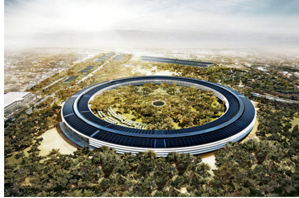
8.14 Apple headquarter NY 2011 , by Foster and Partners actually (22. Apr 13) $ 132 Billion pile of cash. A "net-zero energy" campus, the roof of the spaceship holds 700,000 square feet of solar panels, enough to generate 8 megawatts of power. (enough to power roughly 4,000 homes.
